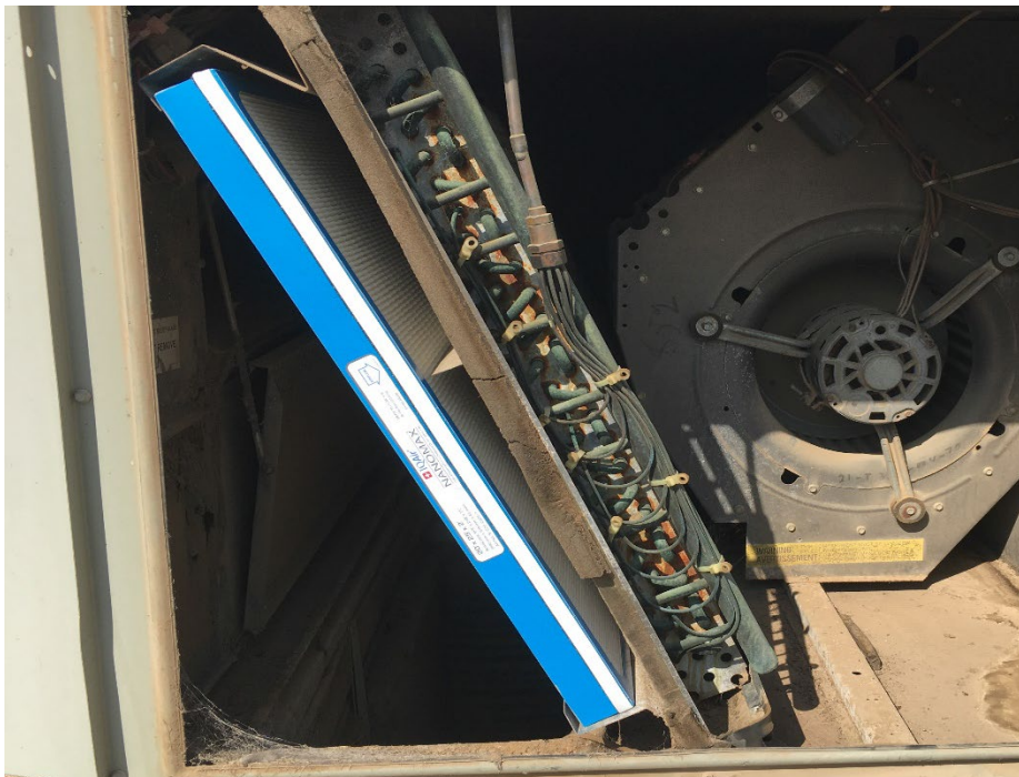
Caption: HVAC unit with IQAir High Performance Filter (Heber School, Heber, CA)
