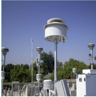
Ambient Air Quality Monitoring
